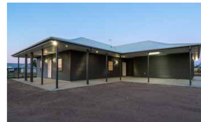
The caretakers' cottage will be perfect for the Hildasid Farm caretaker. The cottage would not have been possible without the support of our construction industry.
